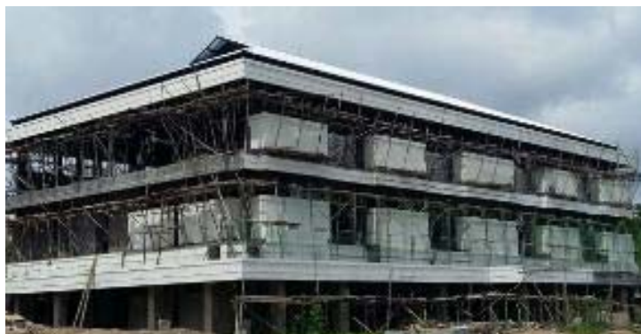
Boarding school works, middle January.
