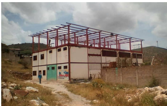
View of the secondary school building, with the extension works in progress.
